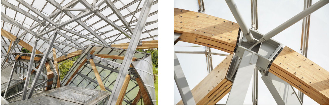
Figure 5.6: A complex 3D steel structure - Fondation Louis Vuitton
