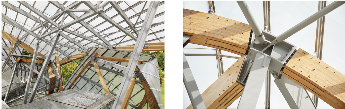
Figure 1.5 – A complex 3D steel structure - Fondation Louis Vuitton
