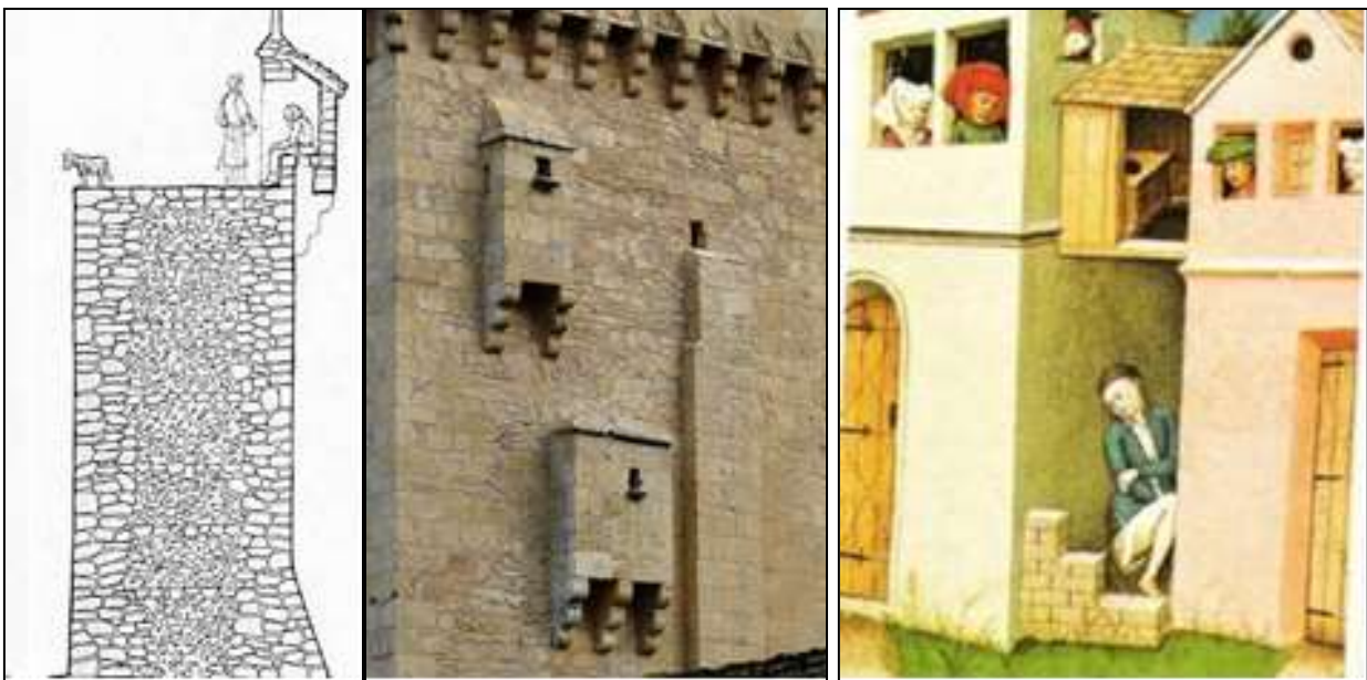
Figure 30 - latrines fixes sans fosse
