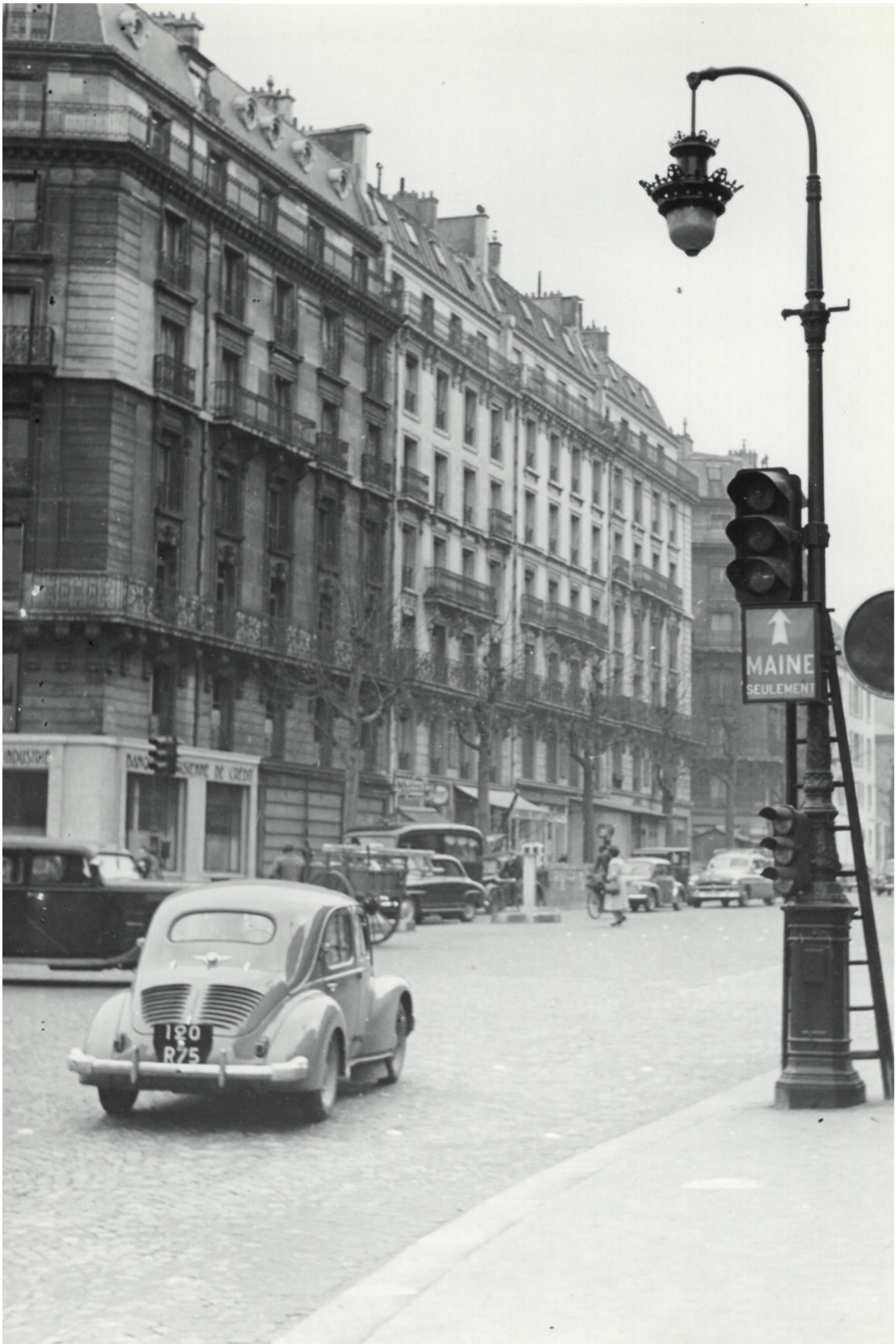
Figure 3.3 – Arrow signal bearing “Maine only” (referring to the Avenue du Maine, in Paris), at the signalized junction between Maine, Montparnasse and Vaugirard arterials. Picture circa 1950, from the Laboratoire des Équipements de la Rue (Paris Streets Assets Laboratory) archives.
