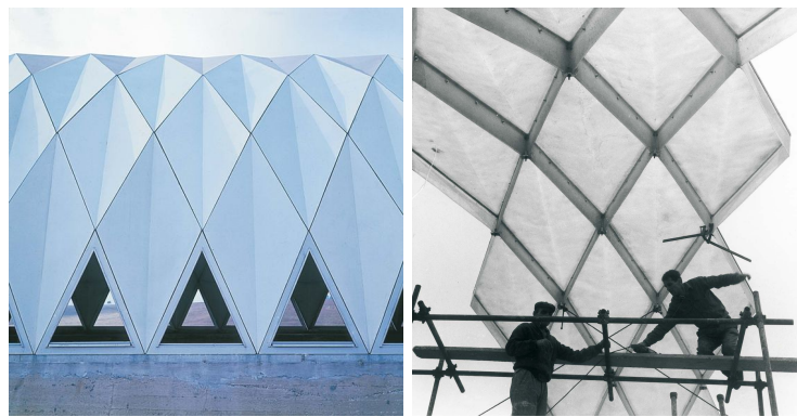
Figure 7.24 – An example of folded plate structures: Sulfur Extraction Facility (arch.: Renzo Piano, retrieved from compositesandarchitecture.com )
