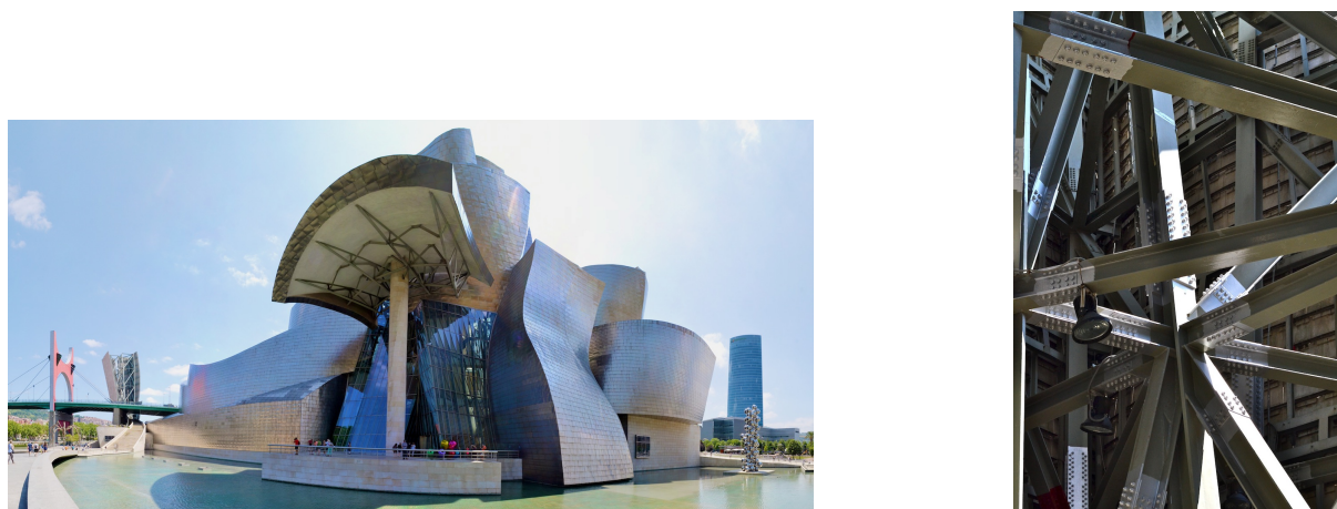
Figure 1.3 – A complex shape can hide an inefficient structure (picture: Romain MESNIL)
