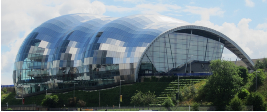
Figure 3.14 – Sage Gateshead Music Centre (architect: Norman Foster): an example of moulding surface covered with planar facets, (picture: Graham Robson, distributed under Creative Commons licence)
