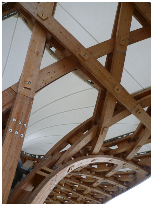
Figure 2.16 – The doubly-curved beams of the Centre Pompidou Metz ( picture: Romain Mesnil )
