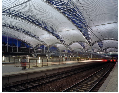
Figure 4.45 – An envelope with varying materials illustrating surface discontinuity ( picture: Samyn and Partners, architects and engineers )
