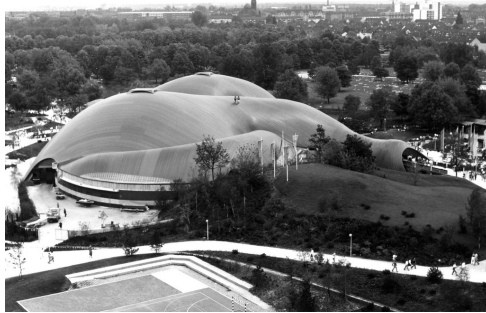
(a) Mannheim Multihalle (archive Frei Otto)
