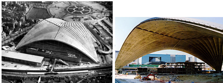
Figure 4.7 – The CNIT: a creased shell designed by Nicolas Esquillan
