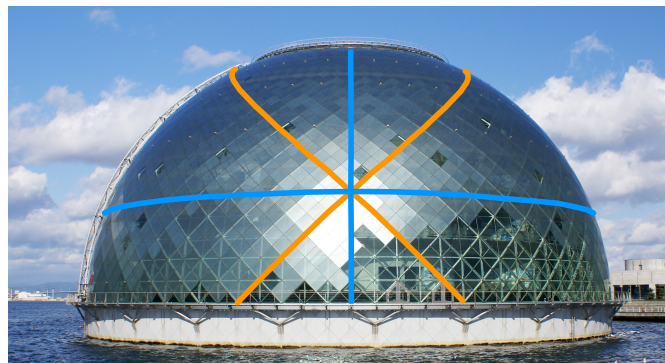
Figure 3.28 – The Maritime Museum of Osaka (architect: Paul Andreu) is meshed with rhumb lines (orange curve) making an angle of 45^\circ with the meridians and parallels (blue) ( picture retrieved on Wikipedia and distributed under a Creative Commons license )
