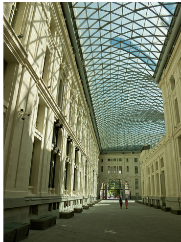
Figure 1.5 – The gridshell covering the courtyard of the Palacio de Comunicaciones ( picture distributed under Creative Commons licence )
