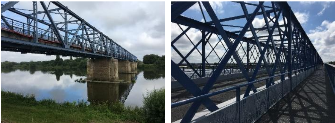
Fig. 1. Haut-Village Bridge (left) and Mauves Bridge (right).
