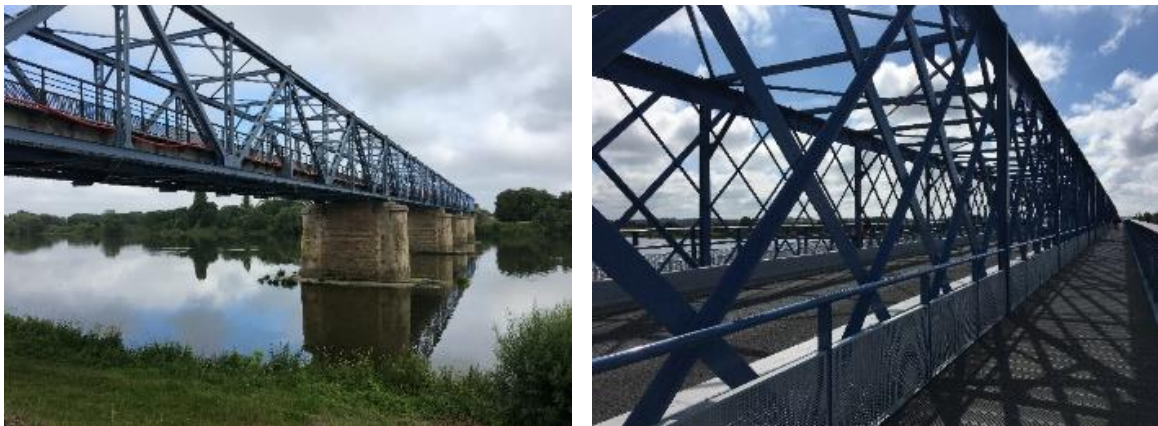
Fig. 1. Haut-Village Bridge (left) and Mauves Bridge (right).
