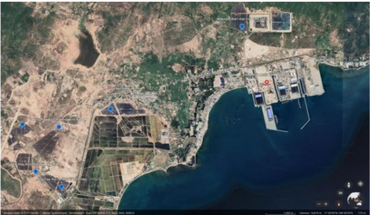
Figure 5: A partially completed coal power center surrounded by new solar farms in Tuy Phong, Bình Thuận, Việt Nam. The red marker shows the empty Vinh Tân 3 project site. Source : Google Earth.
