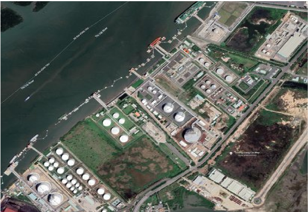
Figure 2: Thi Vai terminal, the first facility to import liquefied natural gas in Vietnam, is due to complete construction in 2022. Source : Google Earth.
