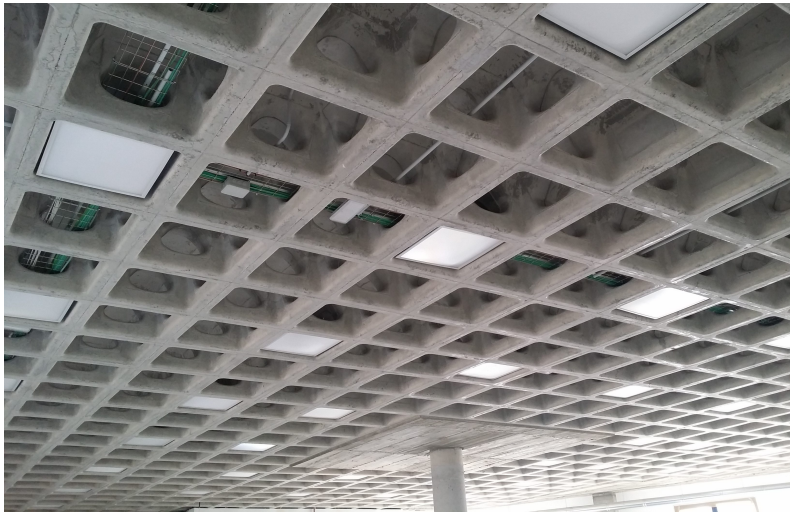
Waffle slab (source: Holedeck )
