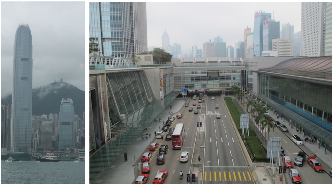
Figure 10. International Finance Center, Hong Kong Central, View of the two skyscrapers skyline and the access to the 'In Town' terminal. Photographies Nathalie Roseau, 2005, 2017.
