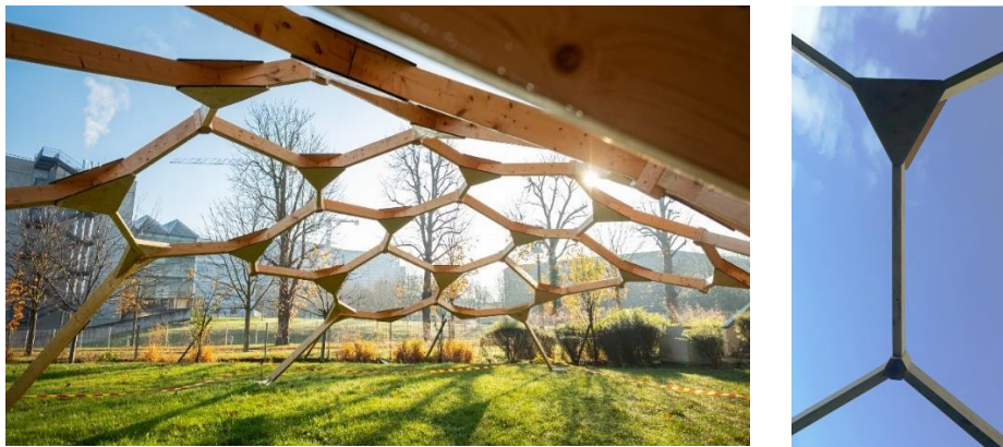
Figure 1: A timber gridshell at Ecole des Ponts, in which many of the properties of Caravel meshes are used to simplify fabrication. In particular, only two types of nodes are used throughout the structure, and beams are cut perpendicularly to the web, which can be done with good precision using low-tech equipment (©Stefano Borghi)
