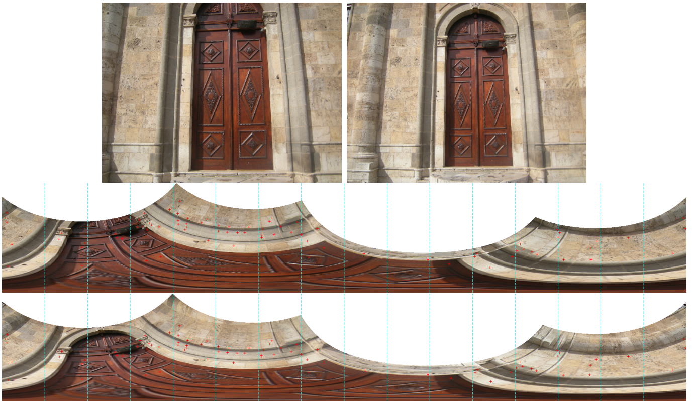
Figure 8: Polar rectification with epipoles inside the image. Rectified images are presented rotated for layout purposes, so that points move vertically.
