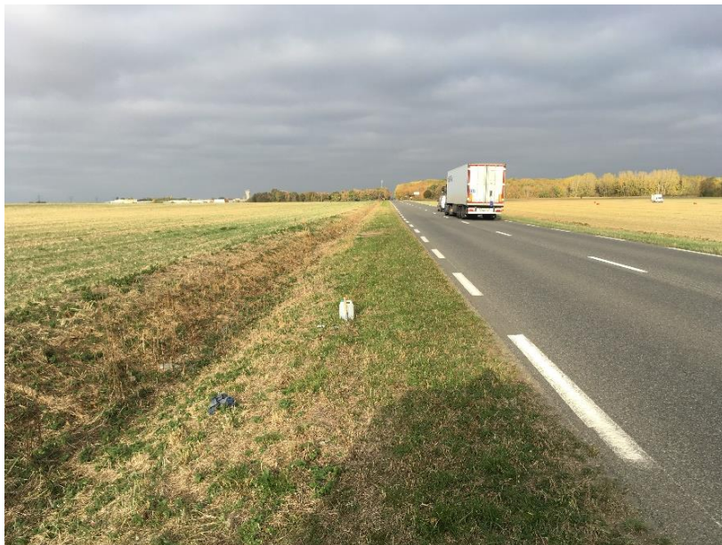
Fig. 1 – Typical French configuration of a vegetated road shoulder followed by a longitudinal ditch.
