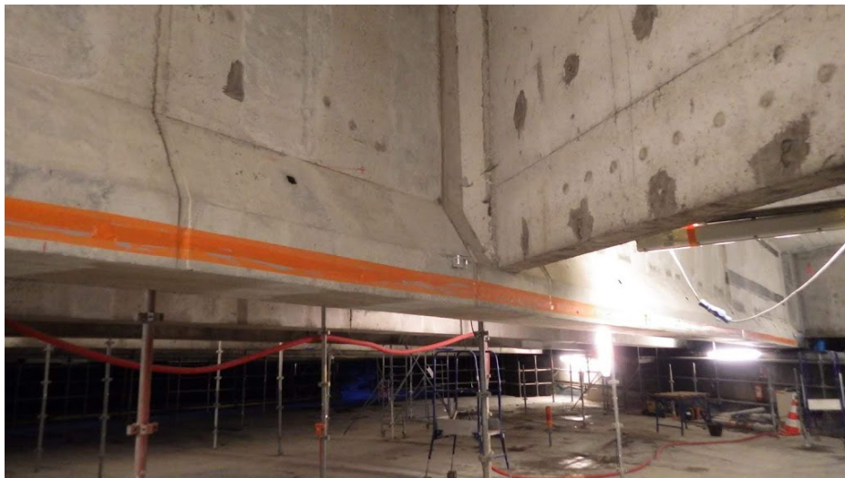
FIG. 8. Girder beam of the Vazeze bridge.
