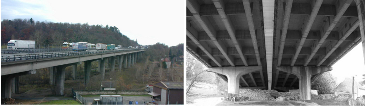
FIG. 1. Roberval bridge and view of its superstructure.
