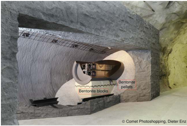
Fig. 1. Nagra concept, based on bentonite blocks and bentonite pellets
