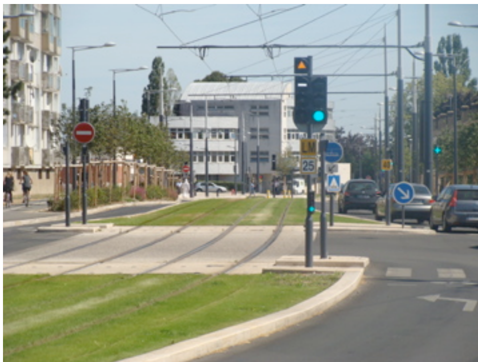
Picture 1: reduced speed across intersections : an illustration along the new line B in Orléans (author: P. Zembri)
