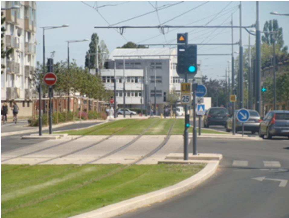
Picture 1: reduced speed across intersections : an illustration along the new line B in Orléans (author: P. Zembri)
