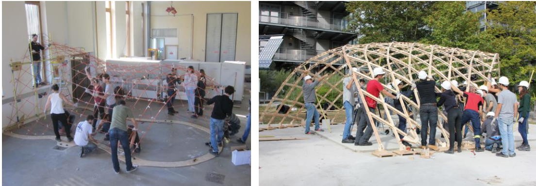
Figure 4: 2015 edition with mock-up like grid (left) and 2016 edition with its full scale wooden grid (right) (photo by courtesy C. Douthe left and S. Lenne right)
