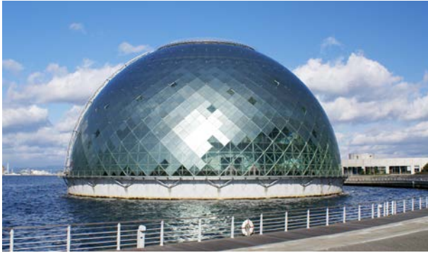
Figure 4: Osaka Maritime Museum: a spiraling pattern following loxodromic curves and creating a PQ-Mesh
