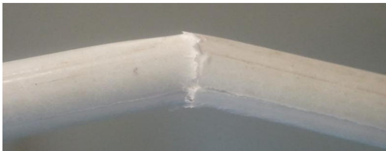
Fig 16. A knee joint type: experimental break of a beam tested in flexion
