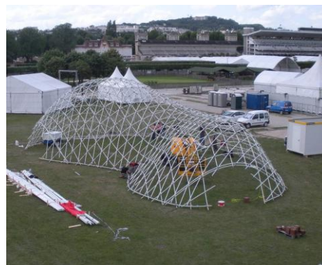
Fig 7. Gridshell anchored and braced
