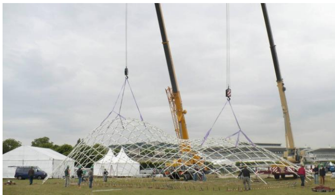
Fig 6. Positioning of the grid with crane
