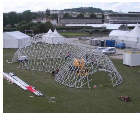
Fig 7. Gridshell anchored and braced
