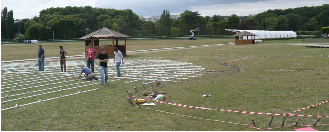
Fig 5. Assembling of the primary flat grid on the ground, near the anchorages
