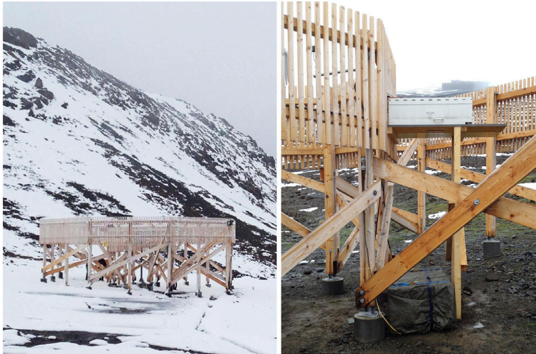
FIG. 1. (left) The DFIR structure and (right) the 2DVD instrument installed on a platform between the two fences near Davos, Switzerland.
