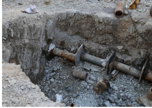
Figure 1. Field test on thin-layer rock masses in dry condition.
