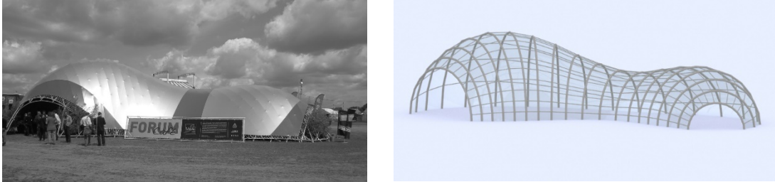
Figure 20: The 'peanut' gridshell of the Solidays forum: built project and interpretation with the inversion of a surface of revolution.
