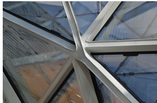
(a) A torsion-free node (inspired by [8]) (b) A node with geometric torsion (picture: Romain Mesnil)
