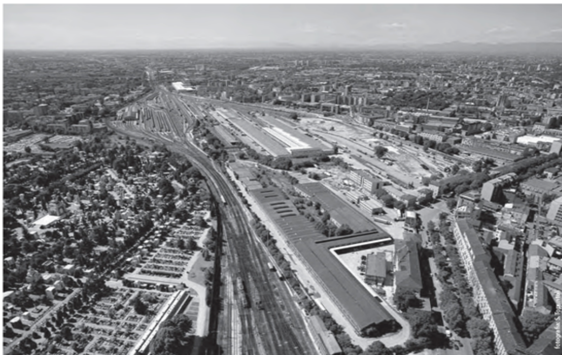
Figure 4: Aerial view of the railway site of Farini in Milan
