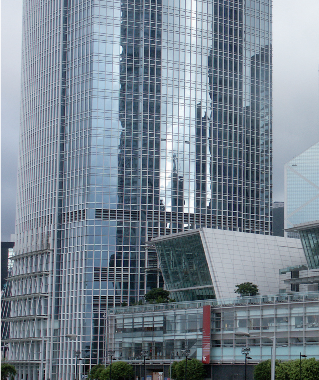
FIG. 8. HONG KONG, VICTORIA ISLAND, CENTRAL AIRPORT EXPRESS STATION E INTERNATIONAL FINANCE CENTER,
