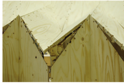
Figure 24. A wood shelter based on a generalization of Miura ori by [117] and the failure mechanism.
