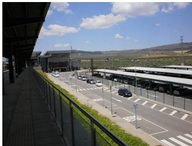
Fig. 4. Antequera-Santa Ana station.
