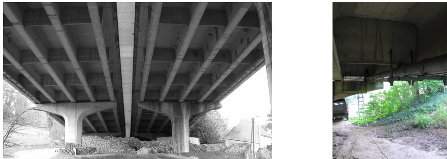
Figure 2. Bridge superstructure (left) and view of a water pipe on girder 1 (right).
