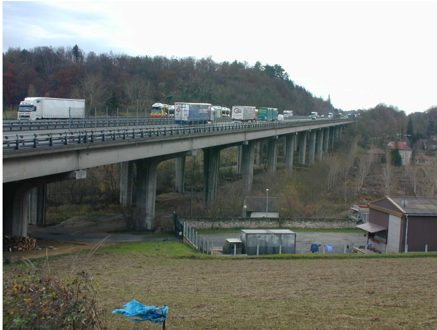
Figure 1. Bridge considered in the study.
