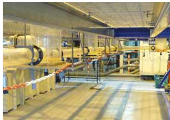
Figure 5b: View from downstream.
