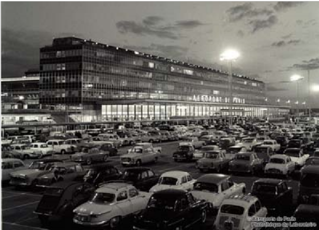
Figure 4. Orly Sud, Paris, The airport Megastructure , 1963.
