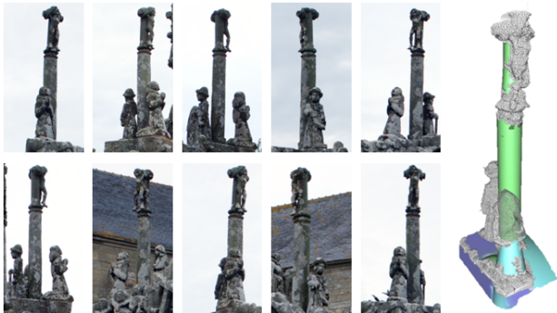
Figure 2. Our hybrid reconstruction with associated multi-view images. Irregular elements such as statues are described by mesh based surfaces whereas regular structures such as columns or walls are modeled by 3D-primitives.
